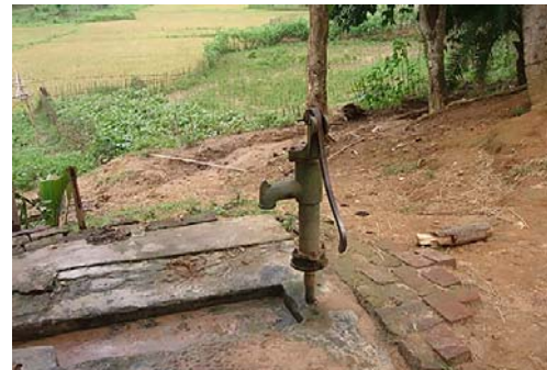
Shallow hand-pump TW used at a school premise in CHT
